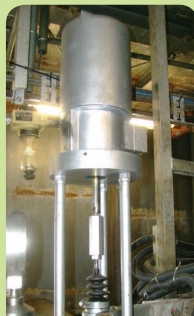
Obsolete pneumatic linear actuator, type Woodward PA 100
