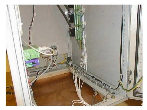
Figure 14-9. Bottom Cable Entry Area
